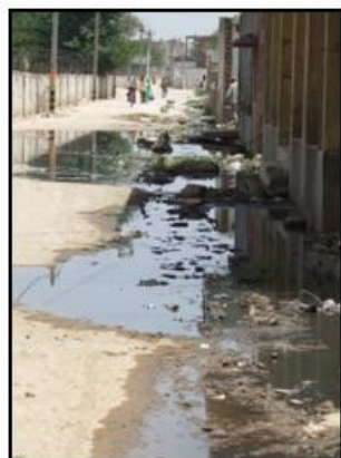
4. LACK OF PROPER DRAINAGE
